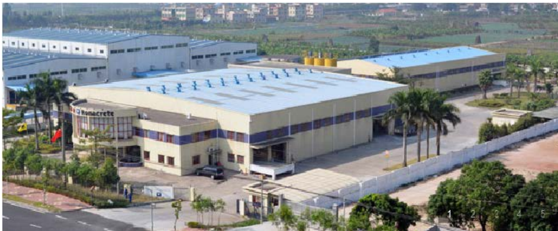
Ronacrete plant in Guangzhou, China
