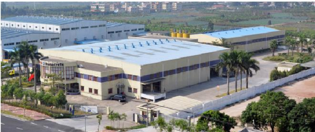
Ronacrete plant in Guangzhou, China
