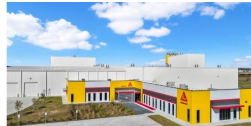
New Houston plant for concrete admixtures and mortar products.
