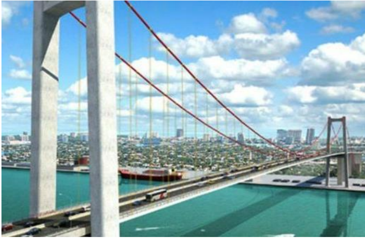
Bridge over Maputo Bay, Mozambique
