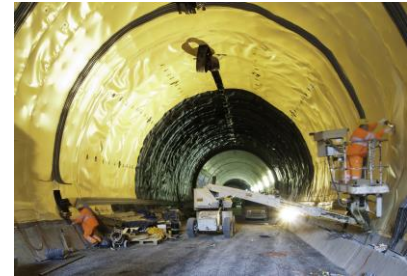
Tunnel projects, Sweden
