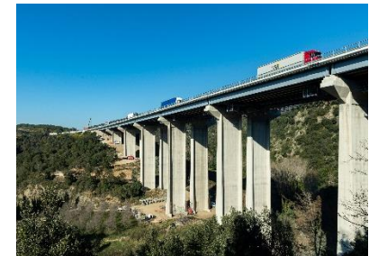
Infrastructure Project, A9, France
