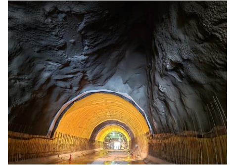
Kra Bao Tunnel, Thailand
