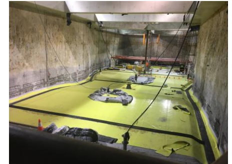
Forrestfield Airport Link, Australia
