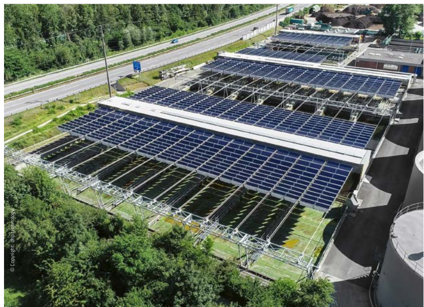
The purification facility clarifiers for the Swiss town of Chur, which are protected and sealed with Sika solutions, have the world's first folding solar roof. Sika made this sustainable concept possible with its fast-curing adhesive and sealant.
